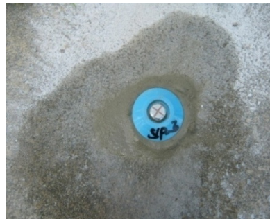
A typical settlement point on pavement
