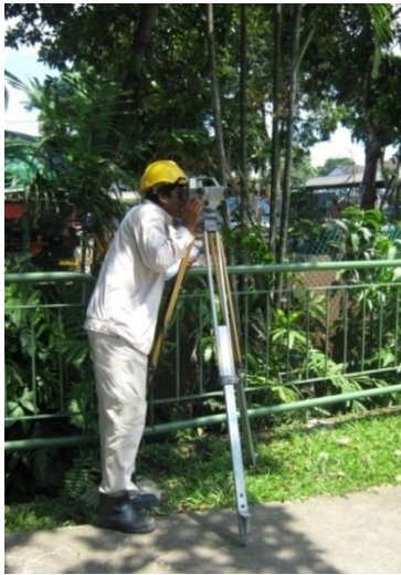
Settlement surveying using digital level
