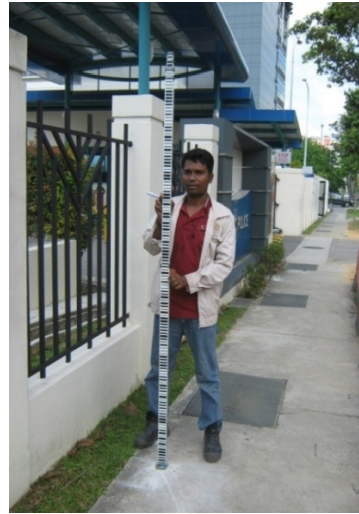
Holding level staff for settlement survey
