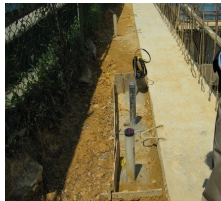
Inclinometer (see pipe in white) installed on a private property
