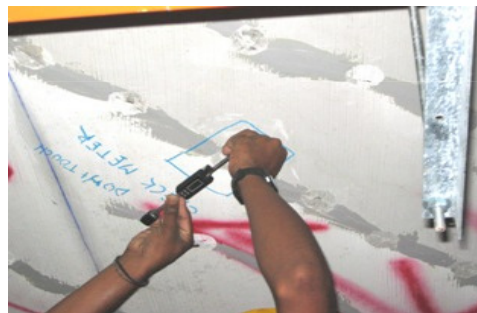
Crack Meter Installation
